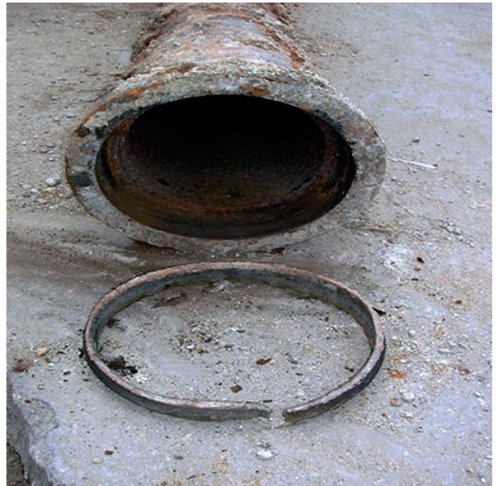
**Fig. 2.** In Philadelphia the joints of the pipes were filled with lead, technique that was also used in Havana.
