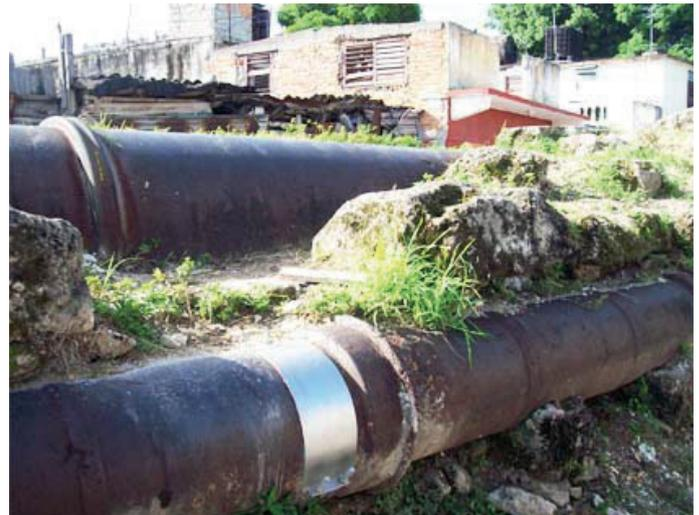
**Fig. 4.** Top to bottom: the iron pipes of Albear (1893) and Fernando VII (1835) showing a repair. The pipes are on top of a wall built to protect them in the street named Resguardo (protection) in Cerro municipality.
